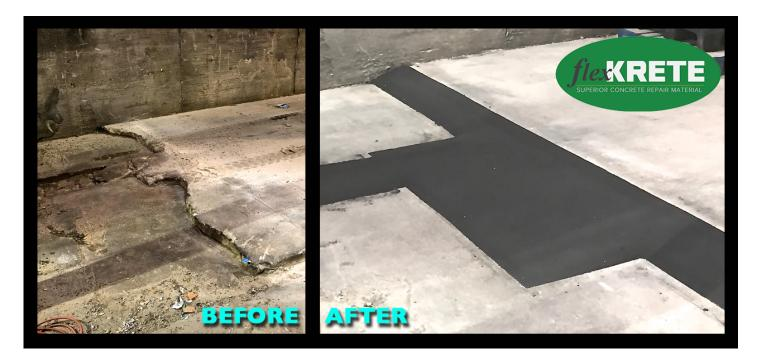
The above image is a great example of how you can repair extremely damaged concrete with multiple issues using a single product. This is a high-traffic area heavy equipment moves 4000-pounds of recycled paper and other materials almost constantly.
